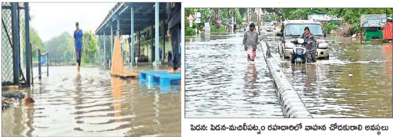
Fig. 13: Water logging in Visakhapatnam and Machilipatnam
